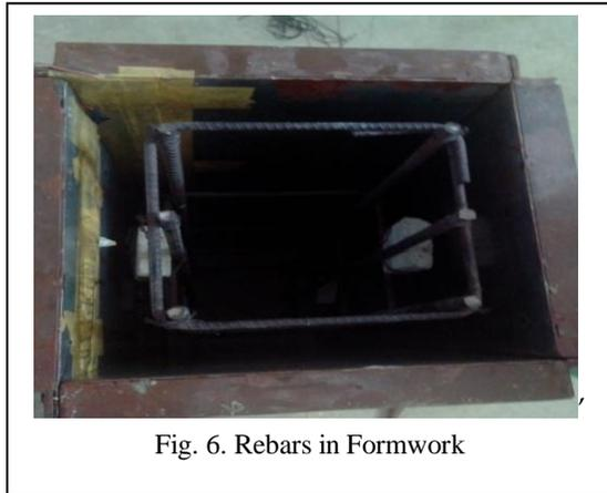
Fig. 6. Rebars in Formwork
