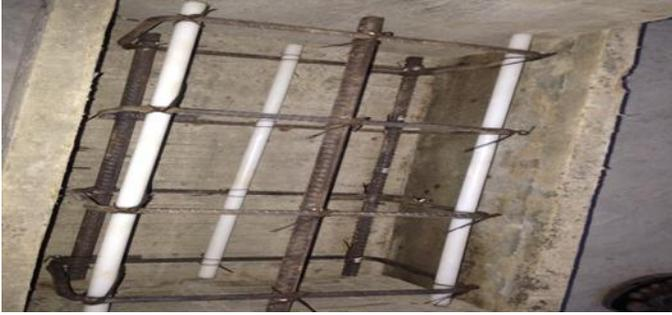
Fig.4 Reinforced with 50% Polypropylene rods
